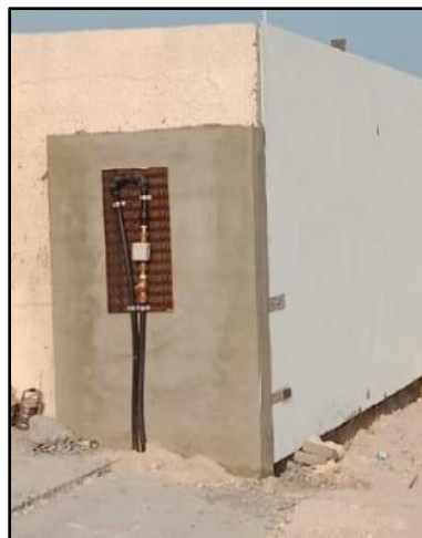
(25mm) Wall Mounted Water Meter on Side Wall
